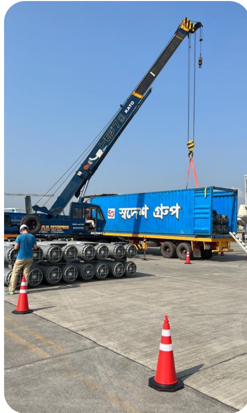
Unloading of Nuclear fuel at Jobsite
